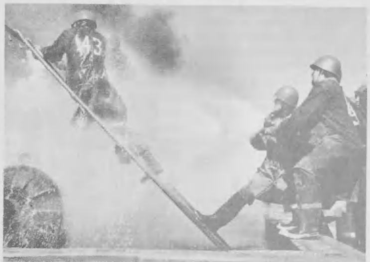
Well protected by fog spray, Marines replace broken ball in overhead leaking flange.
